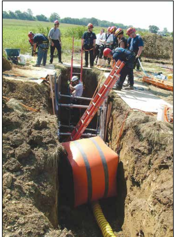
Trench rescue training, KCSRT (Kenosha County Special Rescue Team)
