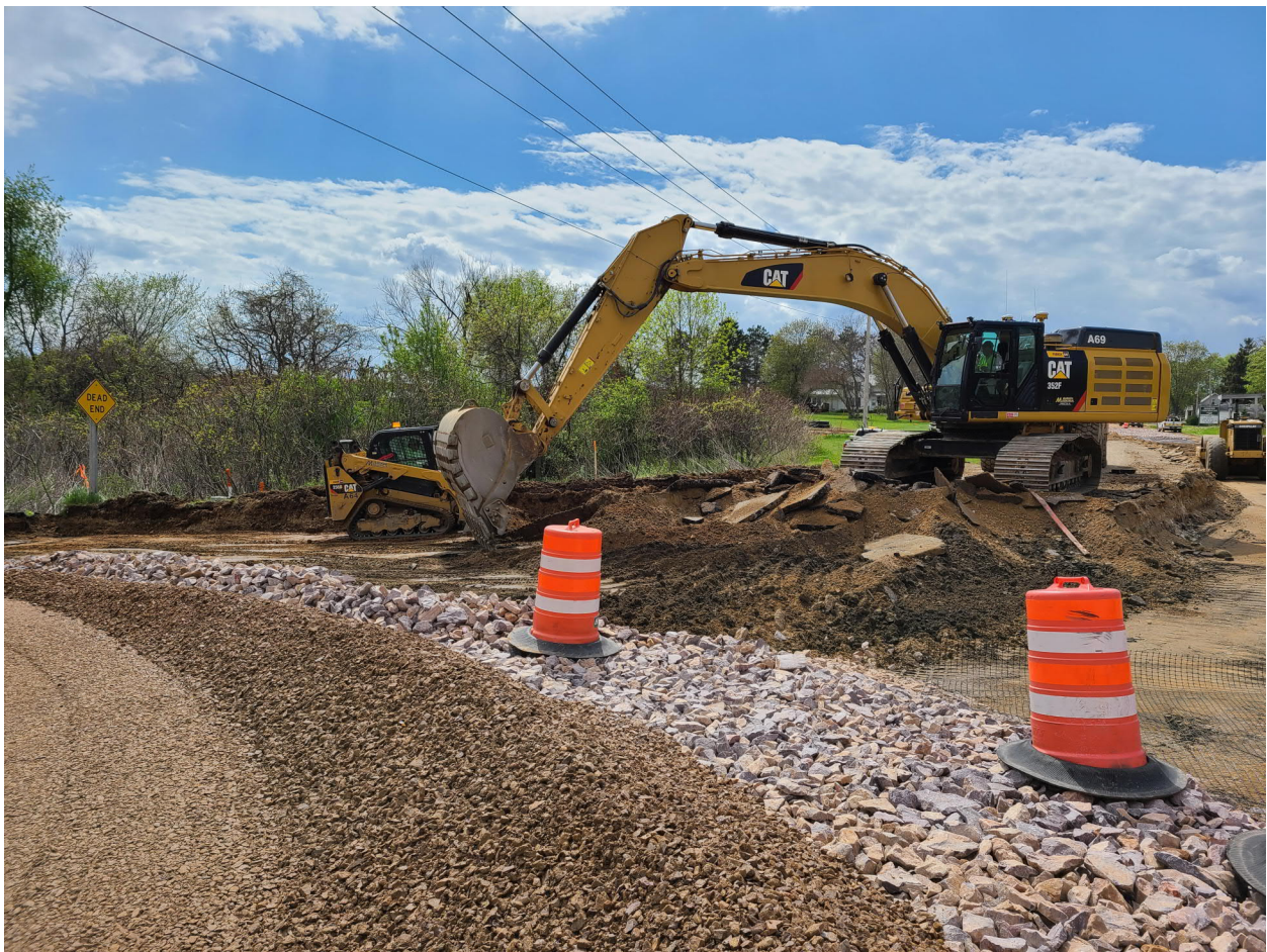
Grading operations at Idlewild Road intersection, (5/6/21)
