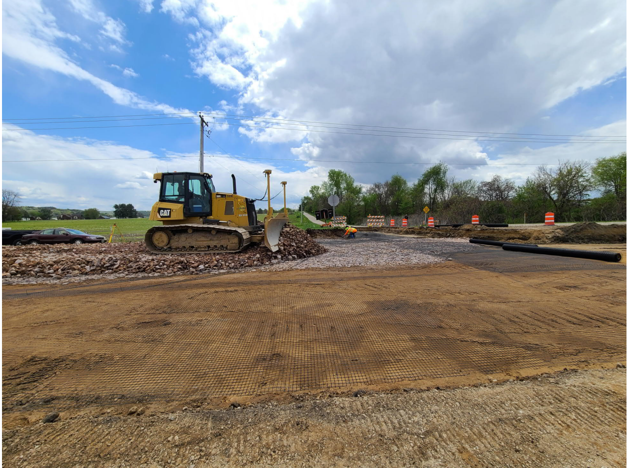
Placing select crushed material at Idlewild Road intersection, (5/6/21)
