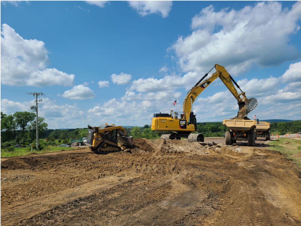
Heavy construction operations grading by Keller Road [N] intersection, (7/01/21)
