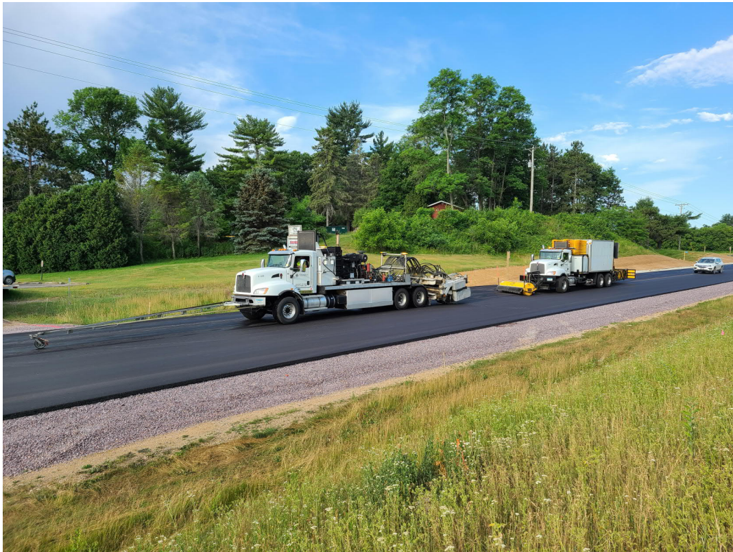
Grinding center line rumble strip near Oak Road intersection, (6/17/21)
