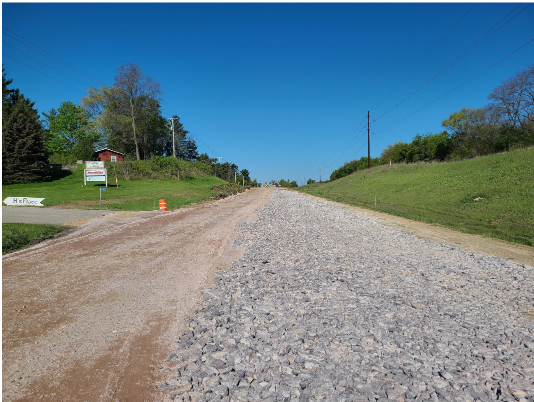
Select crushed material/base aggregate in front of Moon Valley Landing, (5/13/21)
