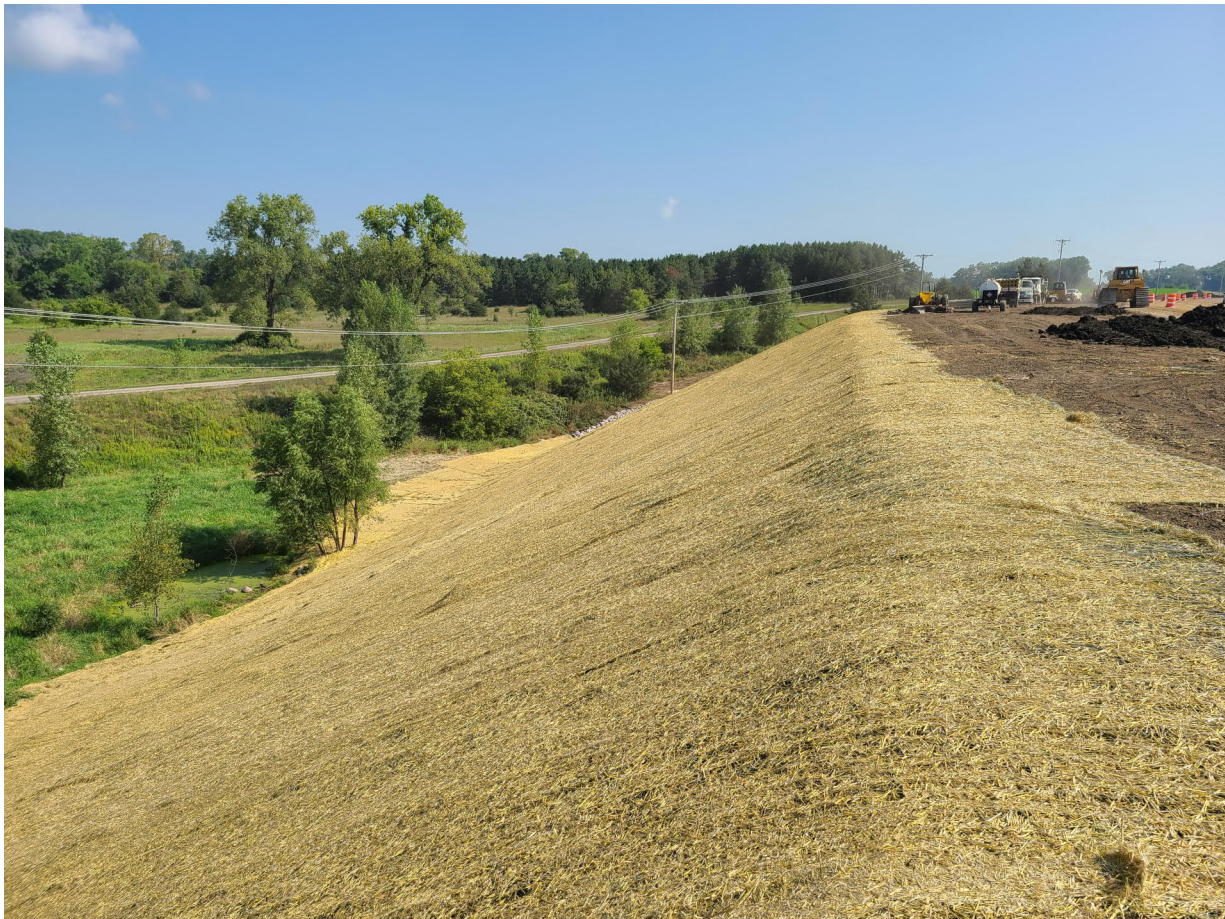
Finished west slope of the large fill section north of Keller Road (N), (8/19/21)
