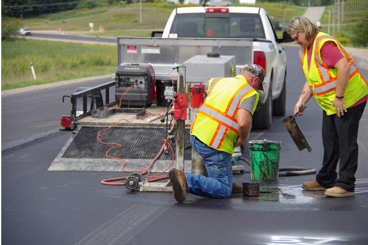
Approaching Goette Road cutting cores to verify the density of the asphalt pavement, (9/2/21)
