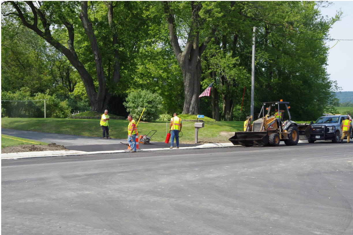
Paving a new asphalt driveway apron west of the Inspiration Drive intersection, (9/2/21)
