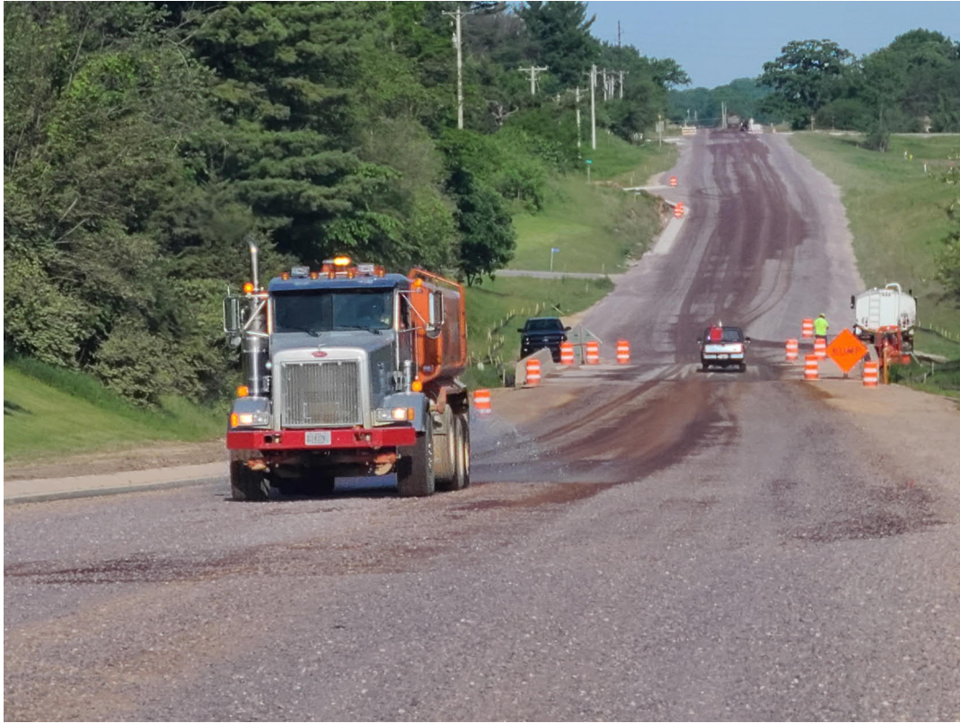
Watering the base aggregate approaching Walleye Lane, (6/3/21)
