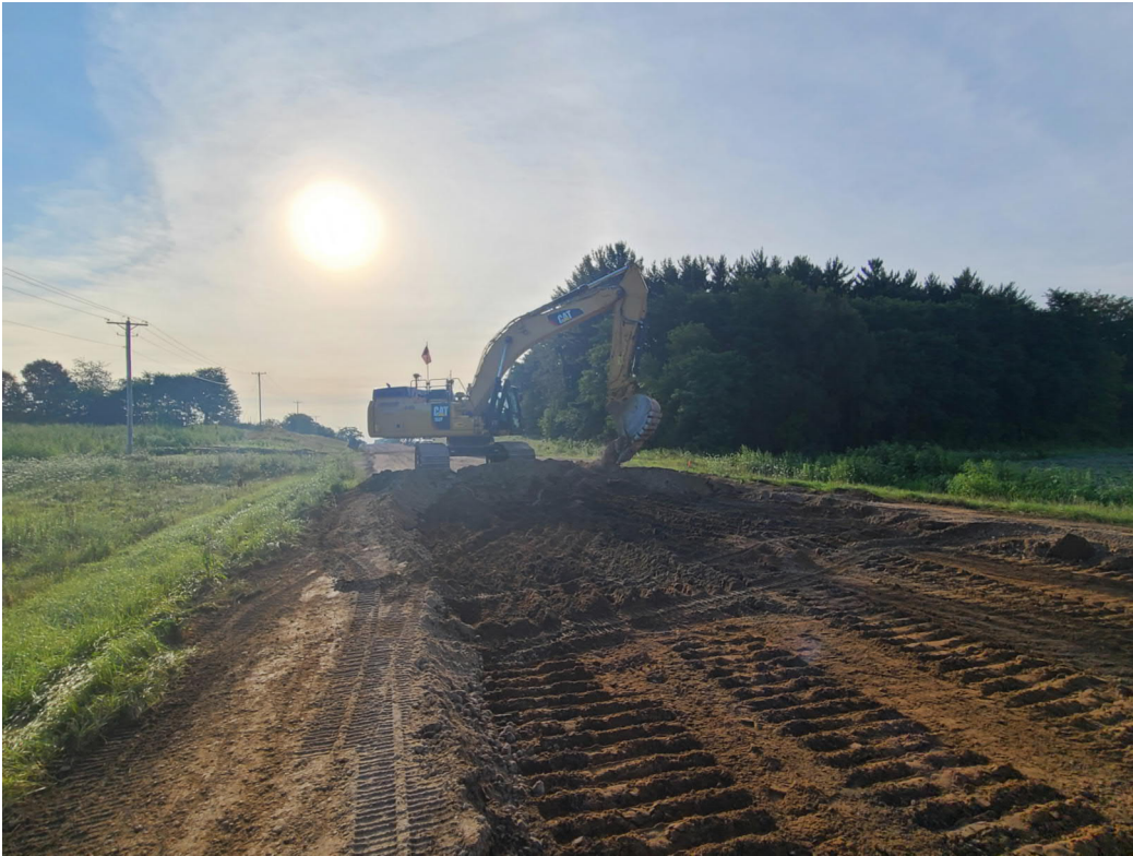
A hot morning, grading towards the connection point west of Eagle Point Rd, (8/12/21)
