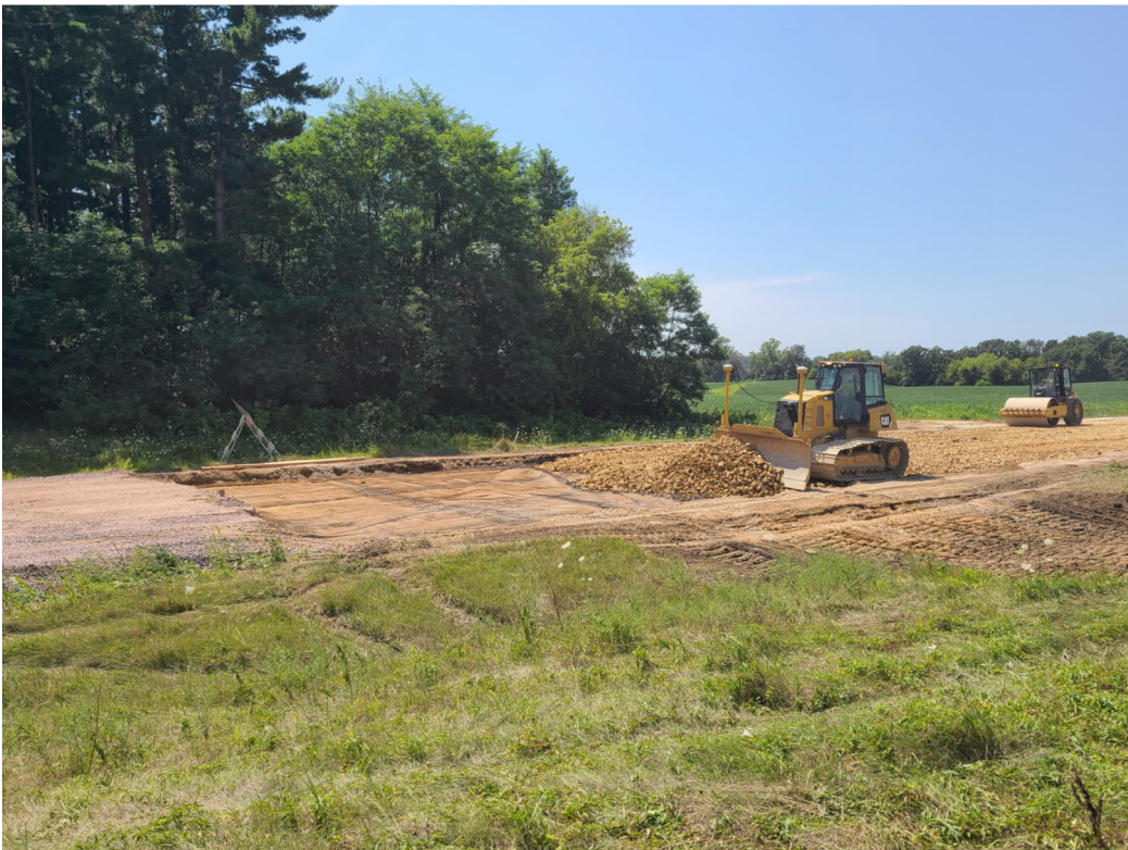
Connecting the roadway with aggregates just west of Eagle Point Road, (8/12/21)
