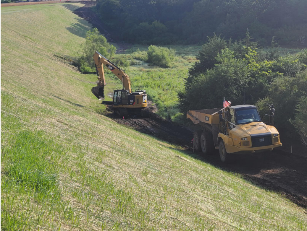
Starting riprap placement in ditch line, large fill area north of Keller Rd [N], (8/12/21)
