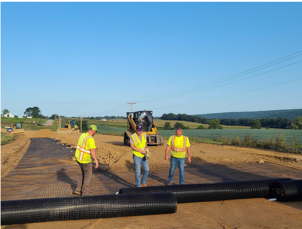
Geogrid installation crew working between Goette Rd & Eagle Point Rd, (8/12/21)
