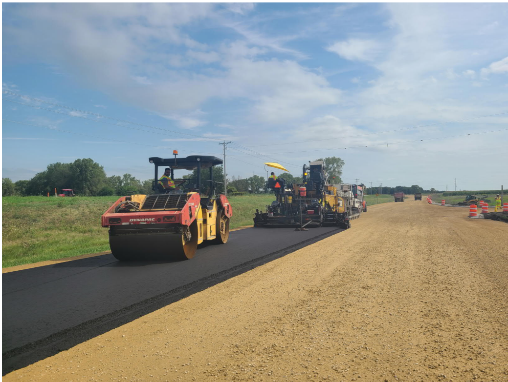
Placing the lower lift of asphalt pavement near the Sunset Drive intersection, (8/25/21)
