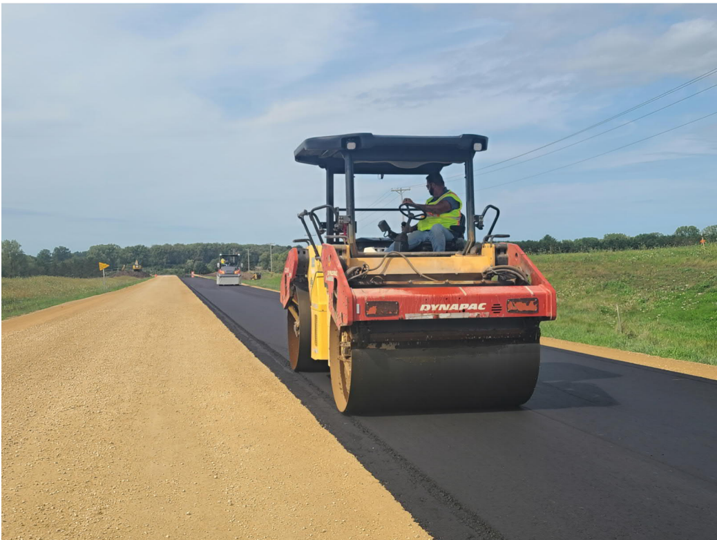
Rollers compacting the lower lift of asphalt pavement south of Sunset Drive, (8/25/21)
