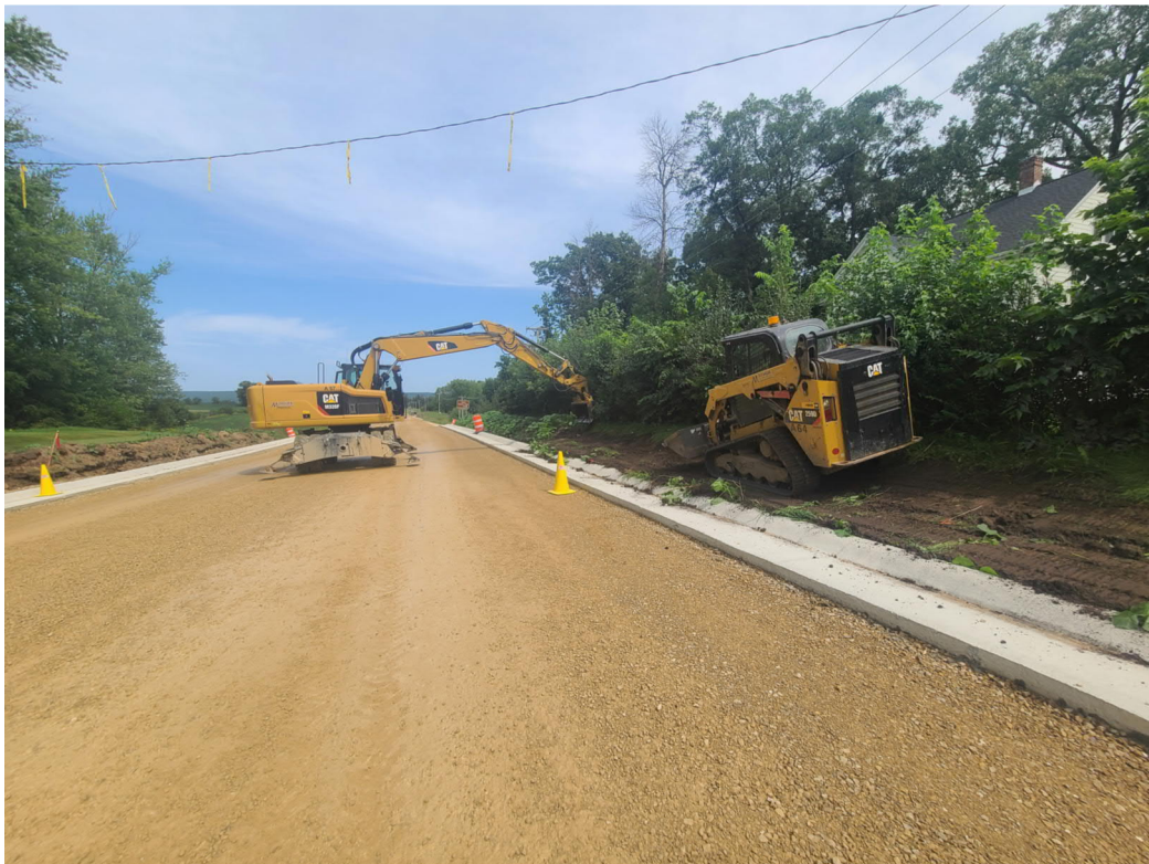
Placing and shaping topsoil behind the curb & gutter by Inspiration Drive, (8/25/21)
