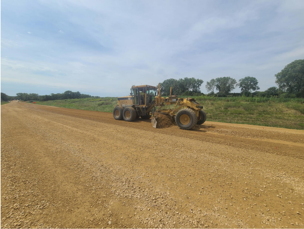
Base aggregate placing and shaping north of Kilpatrick Point Drive, (8/25/21)
