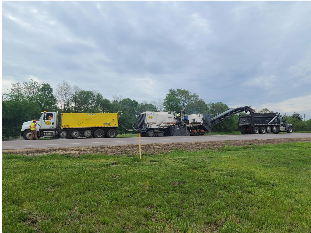
Milling off asphaltic pavement just south of County Z intersection, (5/20/21)
