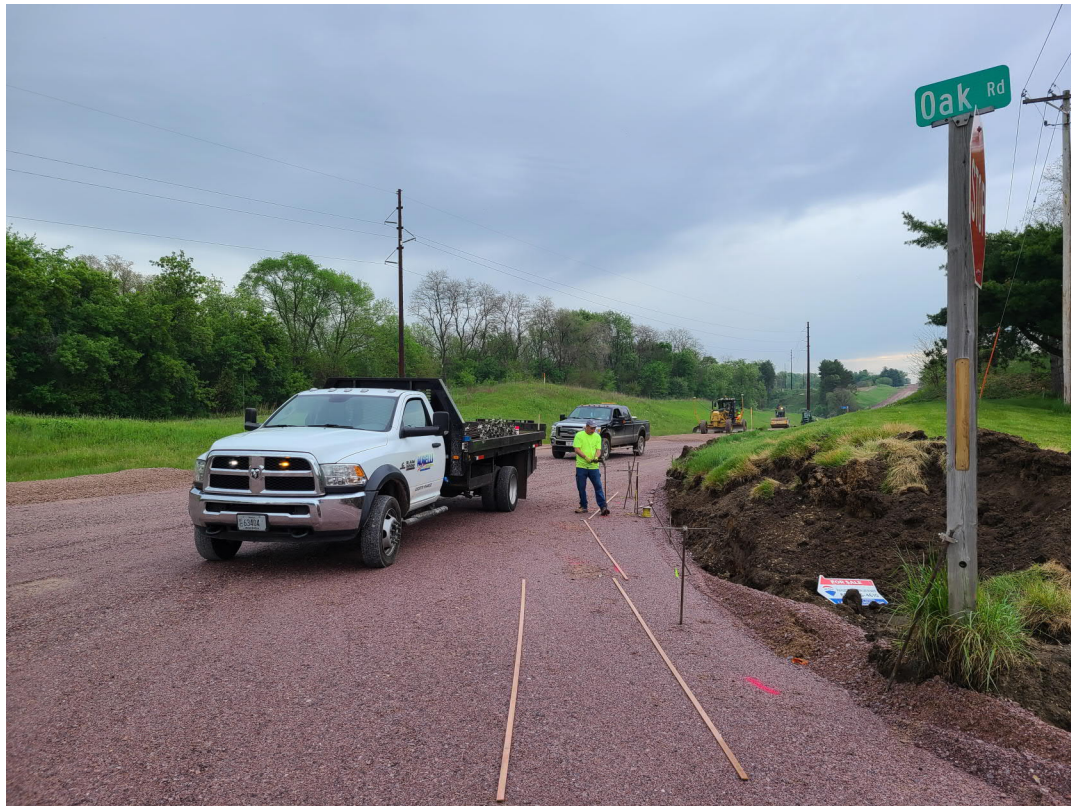
Setting radius slats for curb & gutter placement at Oak Road intersection, (5/20/21)
