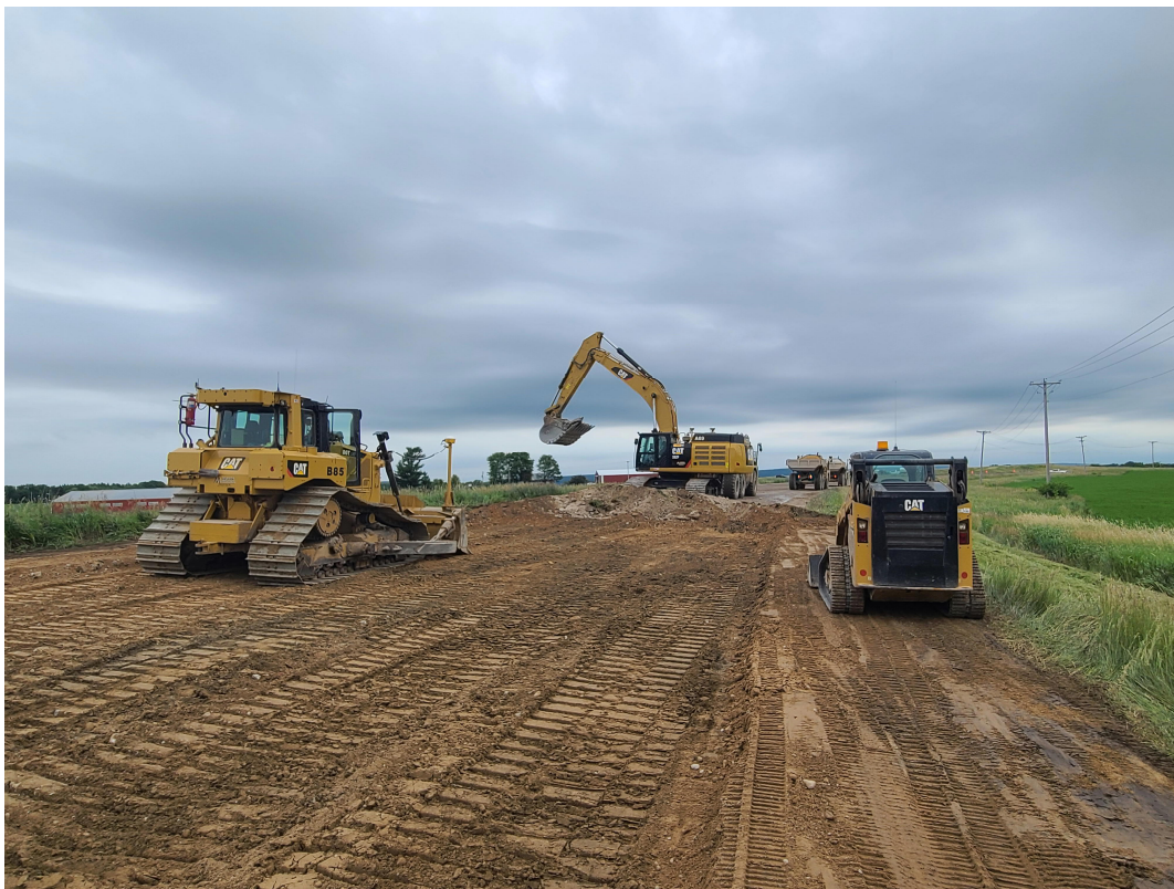
Grading operations digging towards Keller Road [S] intersection, (6/24/21)
