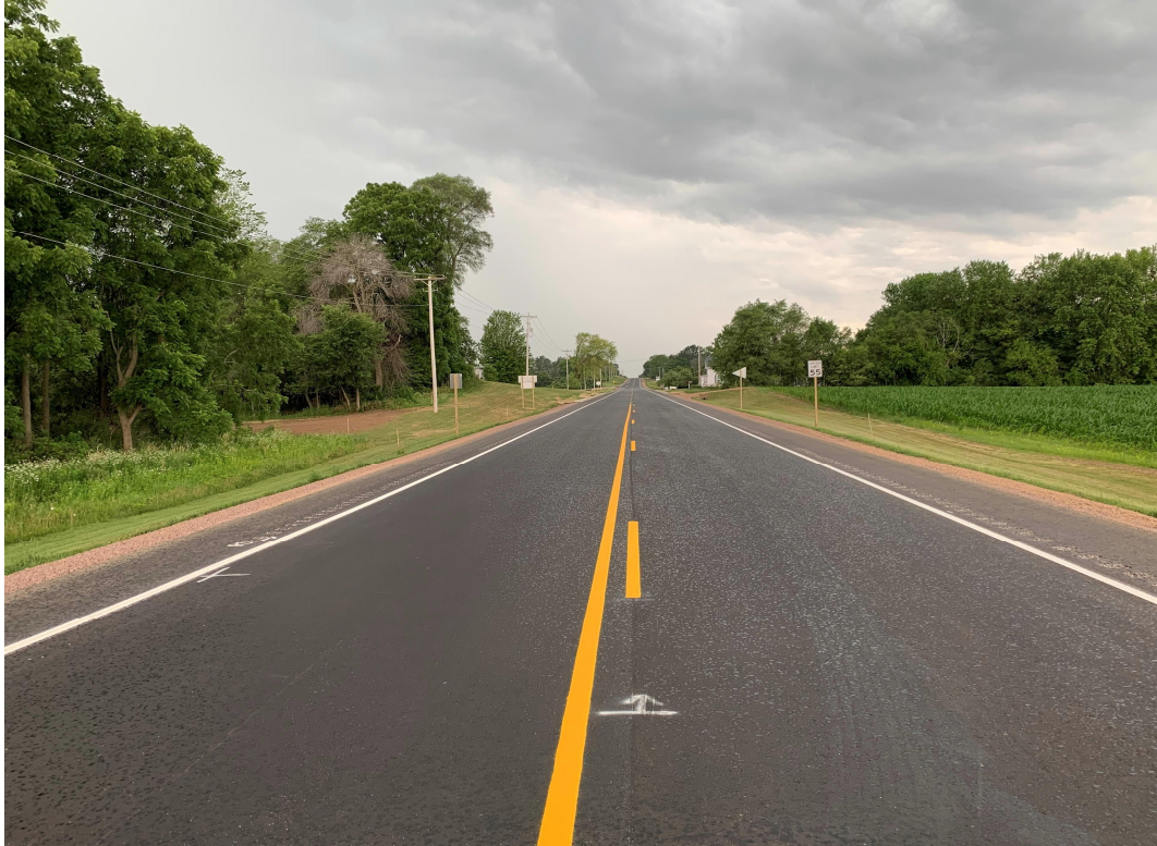
Rain on the recently opened WIS 113 section of the highway, (6/24/21)
