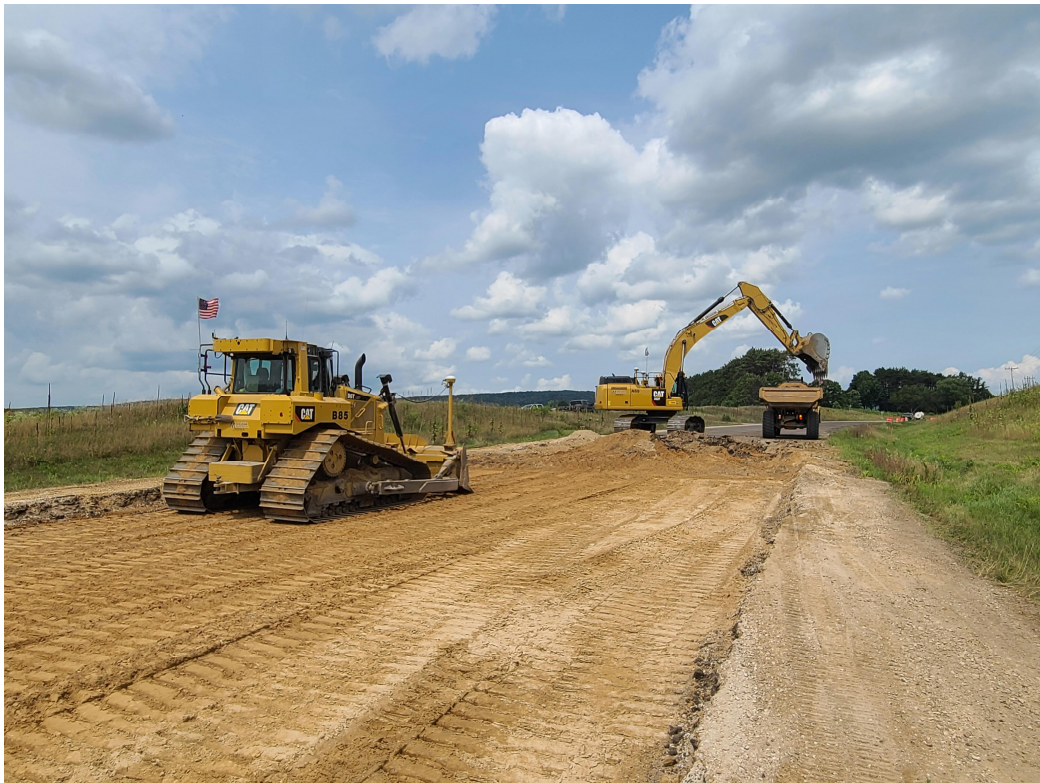
Heavy construction operations grading northward towards Goette Road, (8/05/21)
