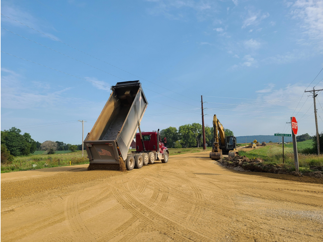
Spreading additional base aggregate in front of Weigands Bay [N] Road, (8/05/21)
