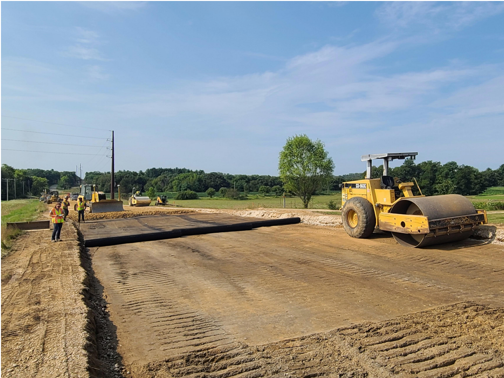
Placing geogrid & select crushed material north of Weigands Bay [N], (8/05/21)
