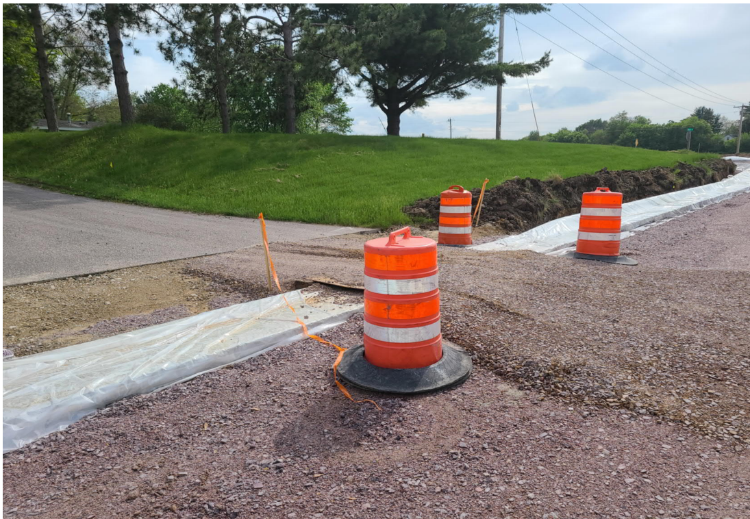
Maintaining driveway access over newly placed concrete curb & gutter, (5/24/21)
