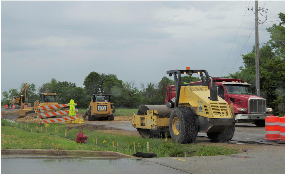
Start of grading and aggregate placement operations by Prairie du Sac, (5/27/21)
