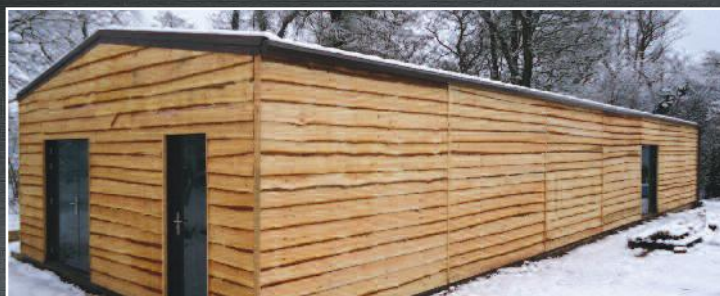
Waney edge boarding system over a fully insulated enclosure as shooting store and ground source heat pump facilities building
