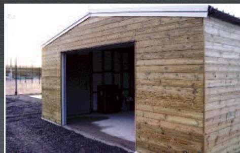
A small facilities building overclad in a tongue and groove boarding
