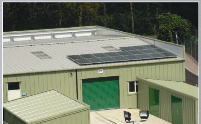
Showroom building with PV generation and two steel framed mono pitch storage buildings
