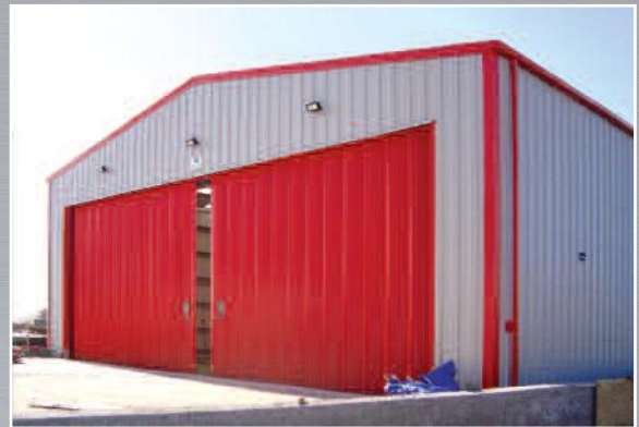
Helicopter hangar building with concertina door system
