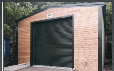
Steel framed workshop with the gable end timber clad to meet planning requirements – neatly bordered by the corner, door opening and barge flashings
