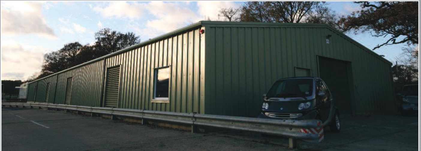
Performance car storage unit with large louver to enable vehicle periodic run ups
