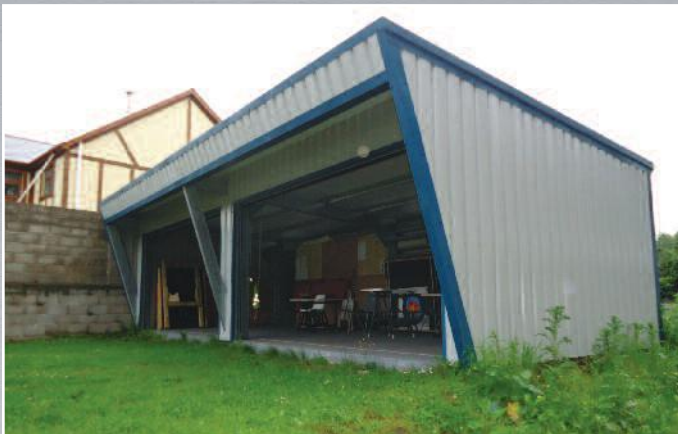
3CB Mono pitch building with overshoot roof for an archery and rifle range
