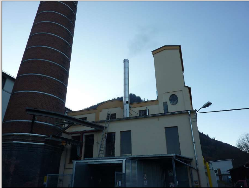
New exhaust system of stainless steel
