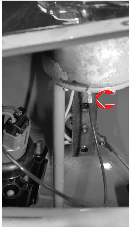
7 The pump's ground (black) wire gets connected to the blade connector (arrow) on the bottom of the fuel sender. It will slip on easily once you have it angled correctly.
