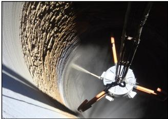
Mancala's remote shaft shotcreting process ensures an efficient and safe non-entry method of applying ground support to shaft walls.
