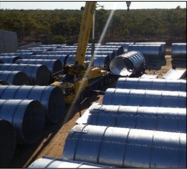
Mancala has adapted and improved the process of using galvanised liners as a non -entry method of ground control for vertical raise bored shafts. The concept uses "modular" liner segments that are bolted together as the installation is lowered into position immediately after the raise borer has completed reaming the shaft.
