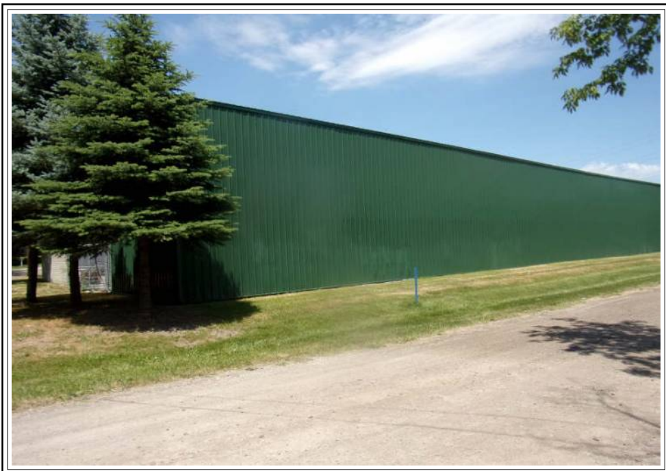
Commercial to the west
