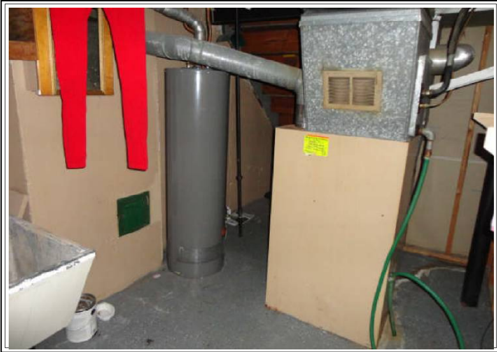
Hot water heater and furnace
