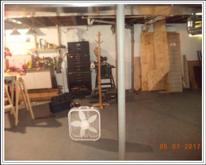
Unfinished basement area
