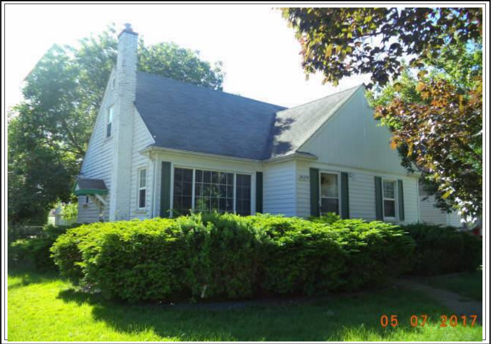
FRONT VIEW OF SUBJECT PROPERTY
