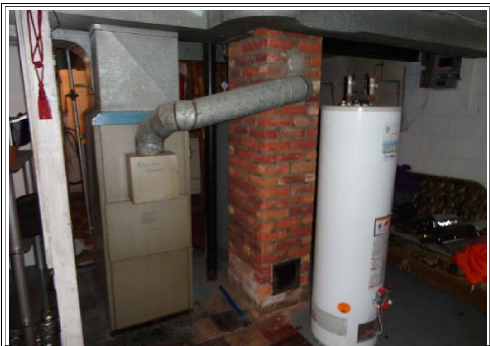
Furnace and hot water heater
