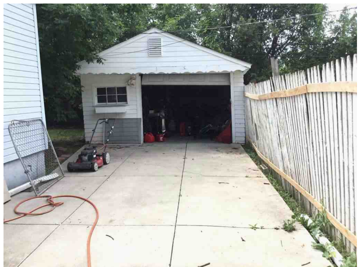
Garage (appears leaning)
