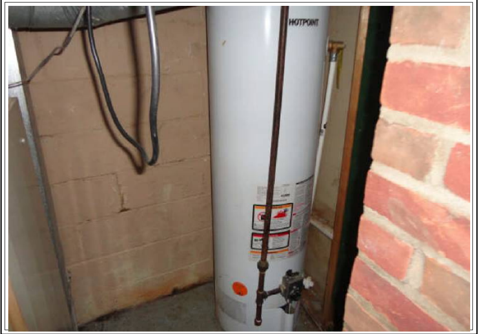
Hot water heater
