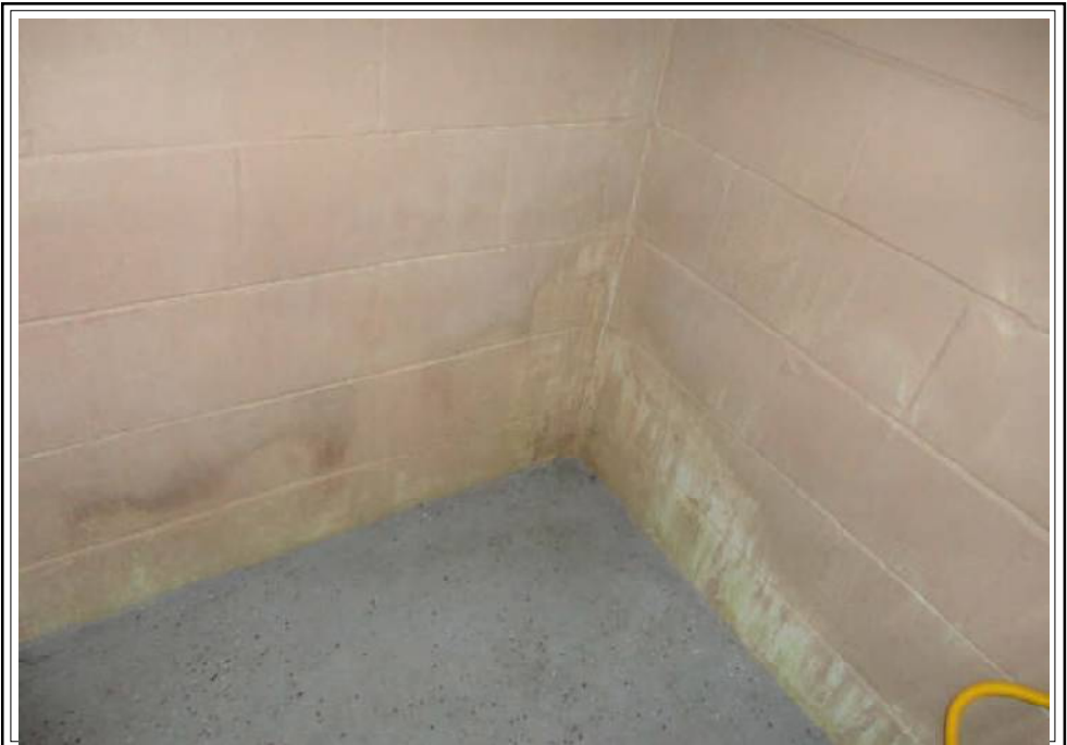
Past water infiltration
