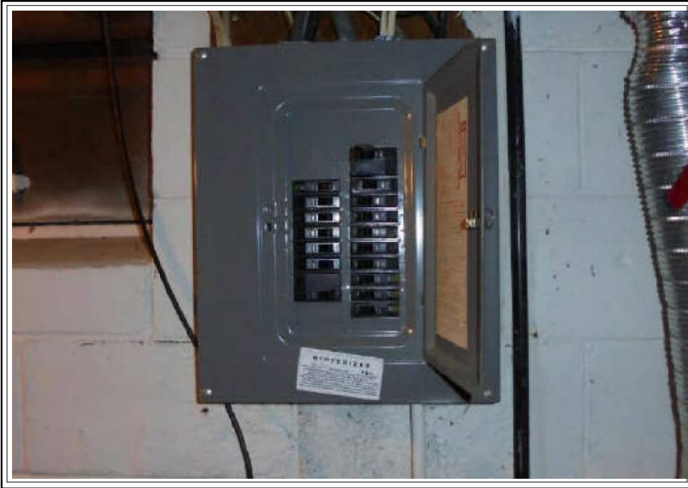
Mechanical Electric Panel
