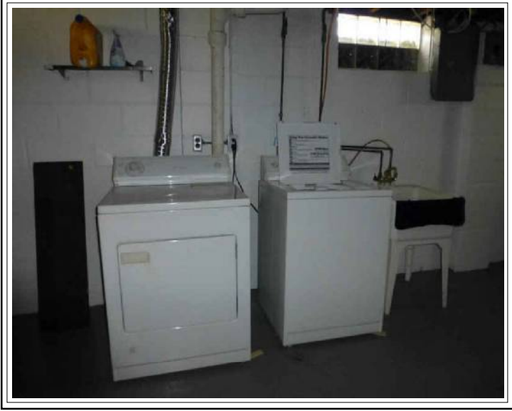
Basement Laundry Area
