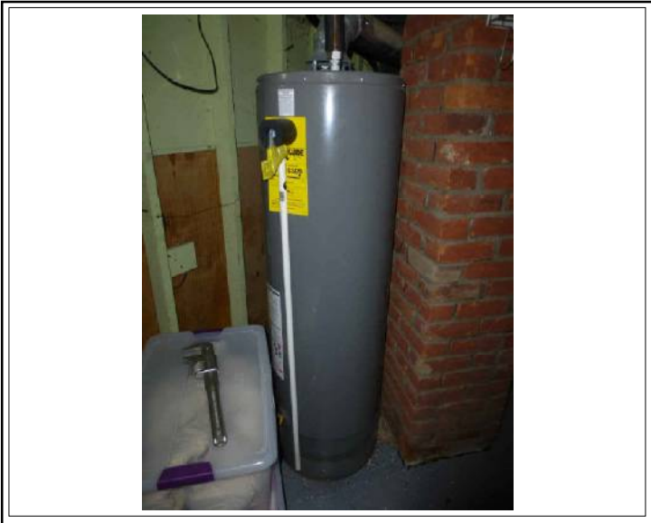
Newer Water Heater
