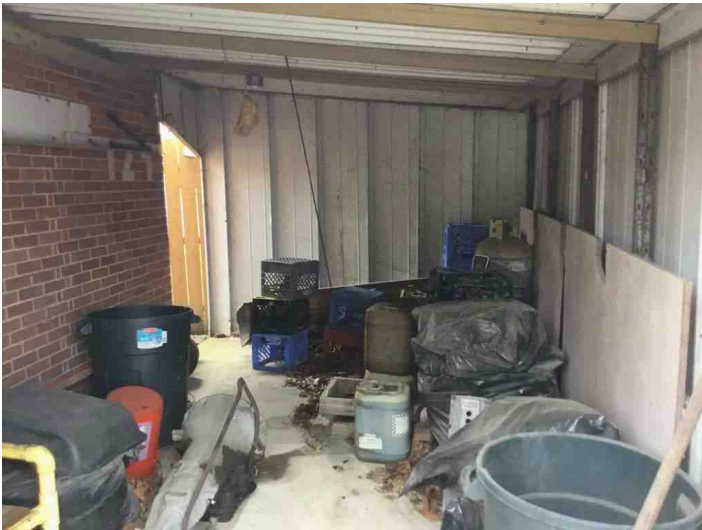
Inside of garage
