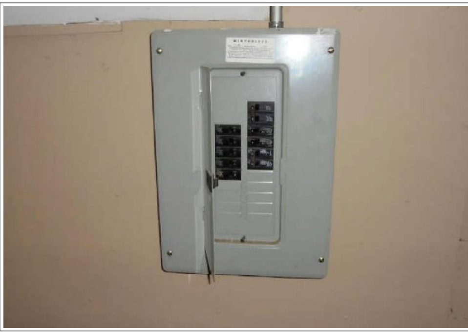
Mechanical Electrical Panel
