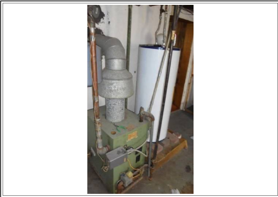
Mechanical boiler/water heater
