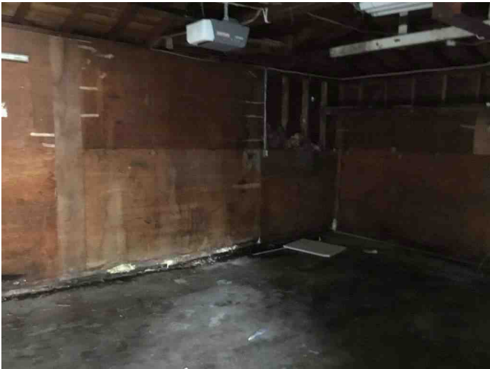
Inside of garage
