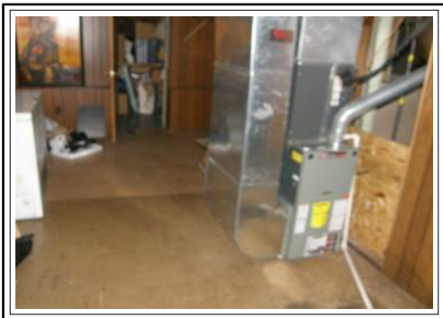
Basement Mechanical Area
