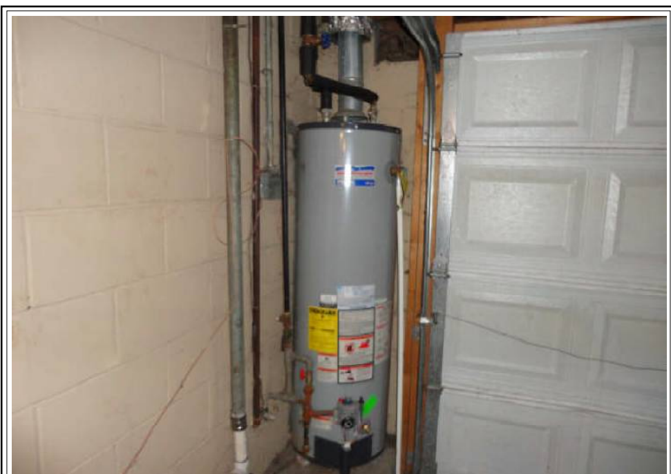
Hot water heater
