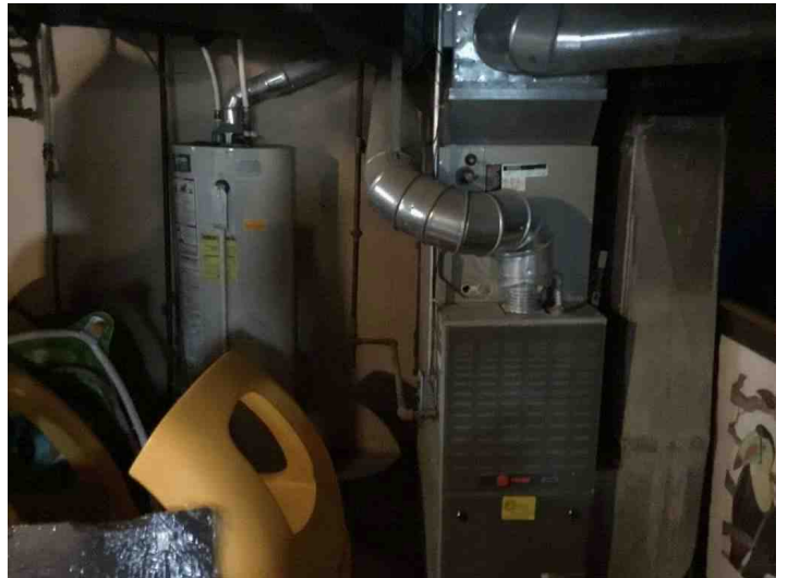
HVAC and HWH
