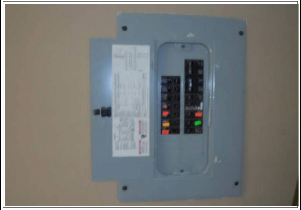
Mechanical Electrical panel
