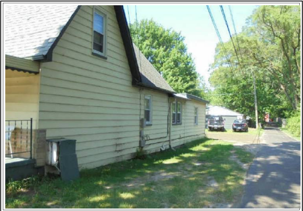
Side view garage
