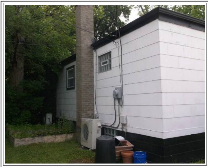
Additional rear view
