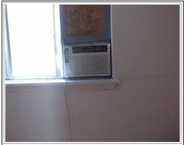
A/C window unit
