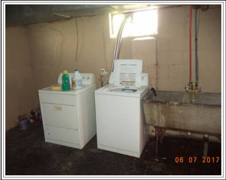
Laundry area in basement
