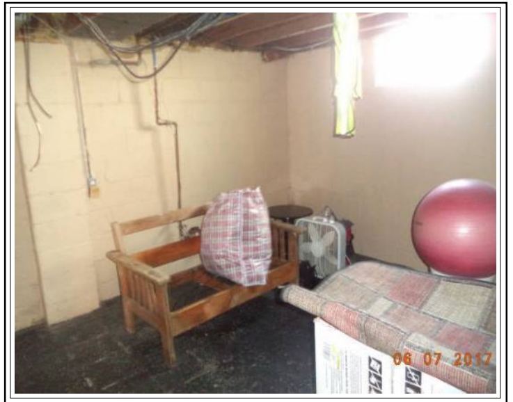
Unfinished basement area
