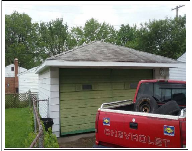
Garage Interior (No health or safety issues noted at time of inspection)
