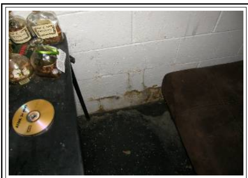
Basement--Possible signs of prior dampness A Foundation Inspection is recommended
