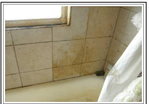
Bathroom Wall and window Possible evidence of mold
