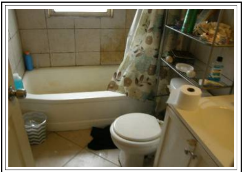
Bathroom.. Possible Mold along walls See Photo Below
