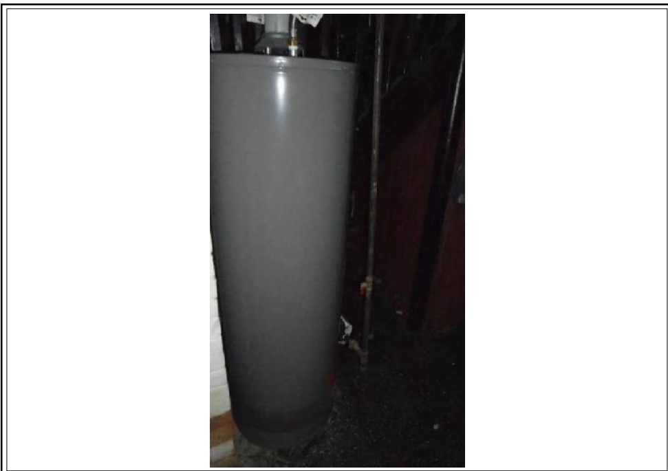
Mechanical Water heater
