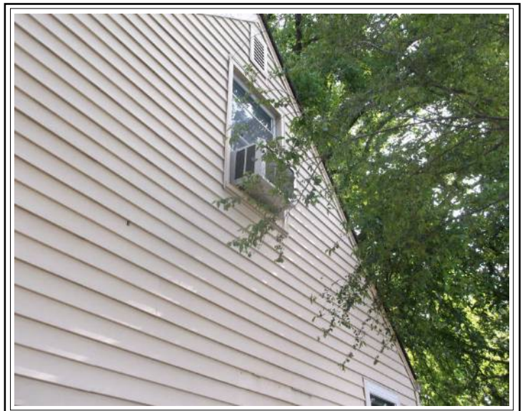
Window A/C unit
