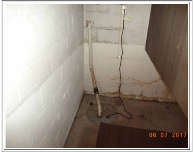
Sump pump Basement
