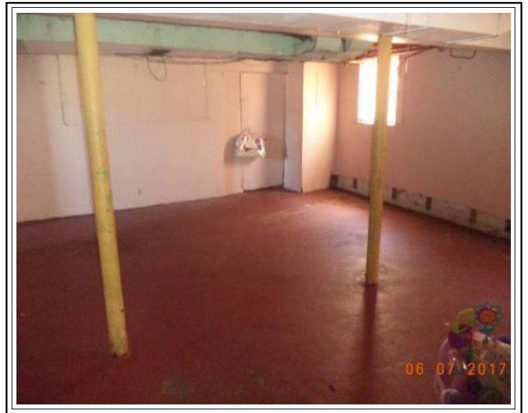
Unfinished basement area
