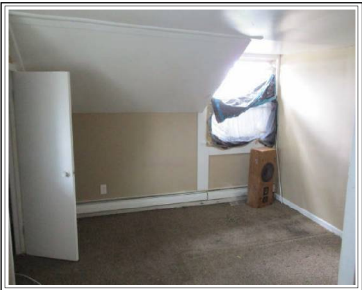
BEDROOM BROKEN WINDOW IN BEDROOM
