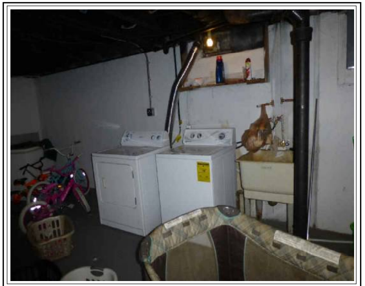
Basement Laundry Area
