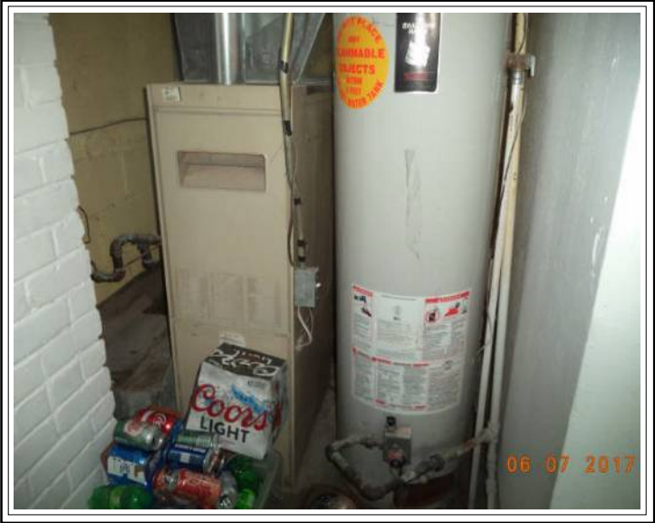
Mechanicals Lower level
