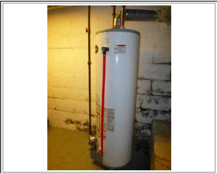
Newer Water Heater
