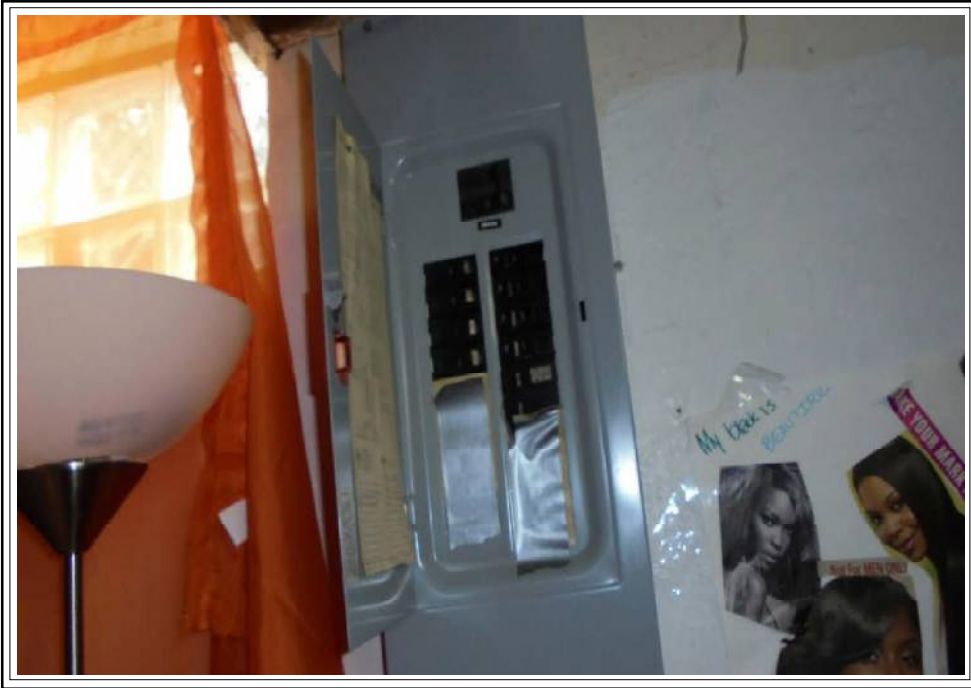
Mechanical Electric Panel
