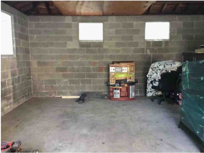
Inside of garage
