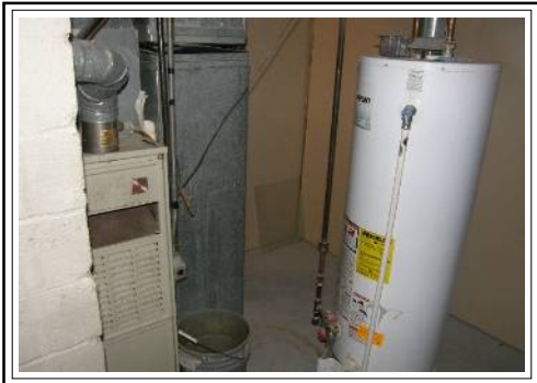
Basement Mechanical Area
