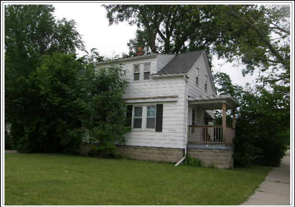
FRONT VIEW OF SUBJECT PROPERTY
