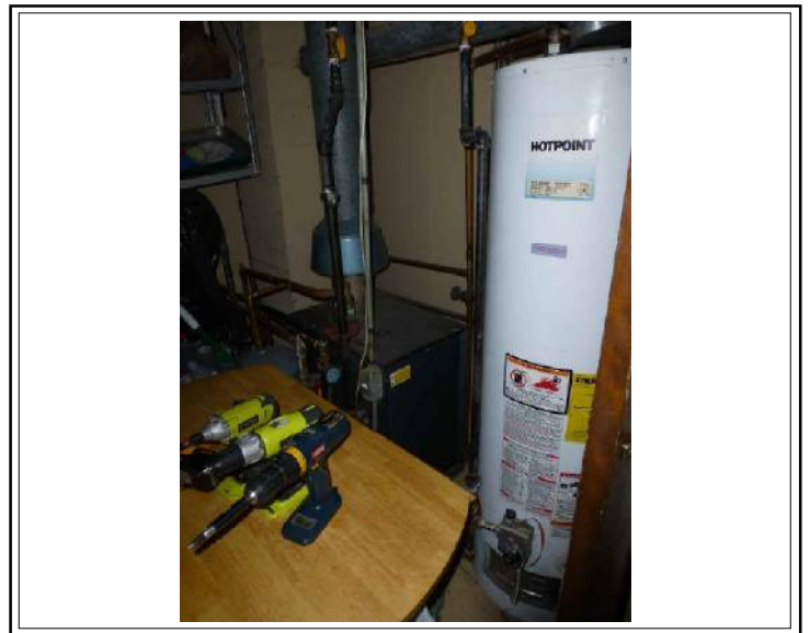
Boiler & Water Heater
